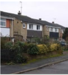
Bad: generic housing infill unrelated to local character and colour palette
