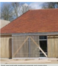
Good: new build with traditional materials and construction.
